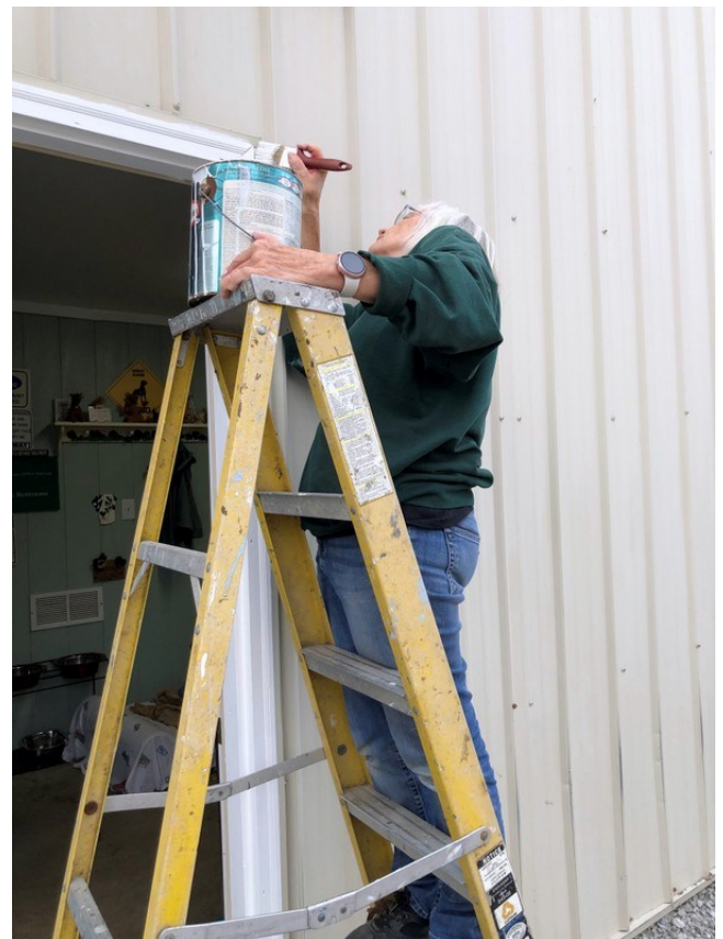
Volunteer Judy Yacks paints trim on the Rescue office doorway.
